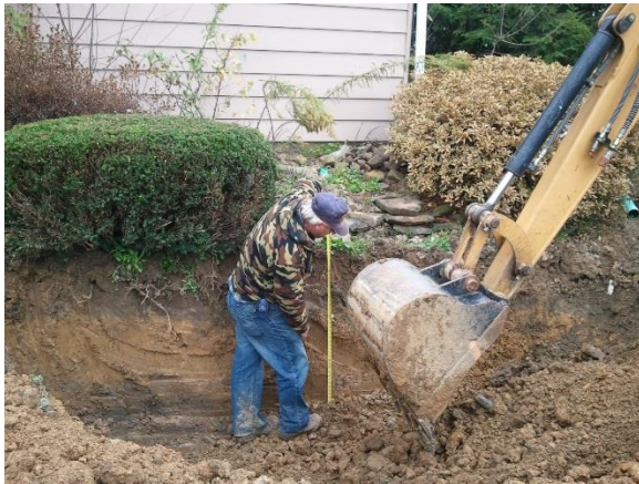
Excavate a drywell at least 10' from foundation
