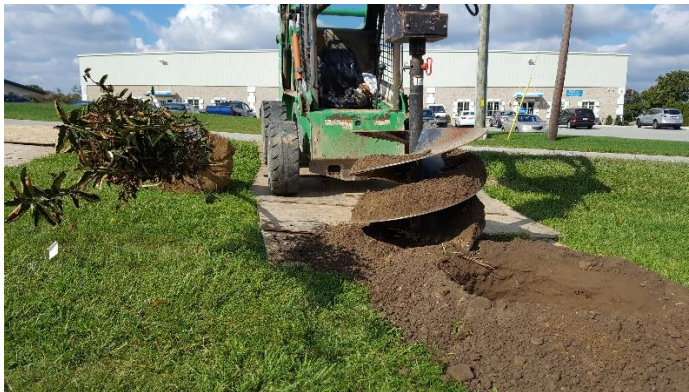
Plywood sheets protect lawn from compaction
