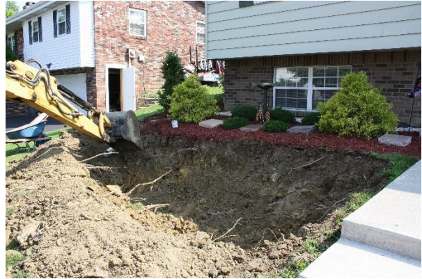
Excavate rain garden at least 10' from foundation
